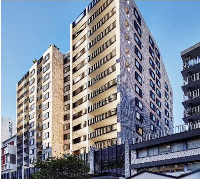
HUTCHINSON BUILDERS Whitton Lane Residential Contract Value: $5,500,000
