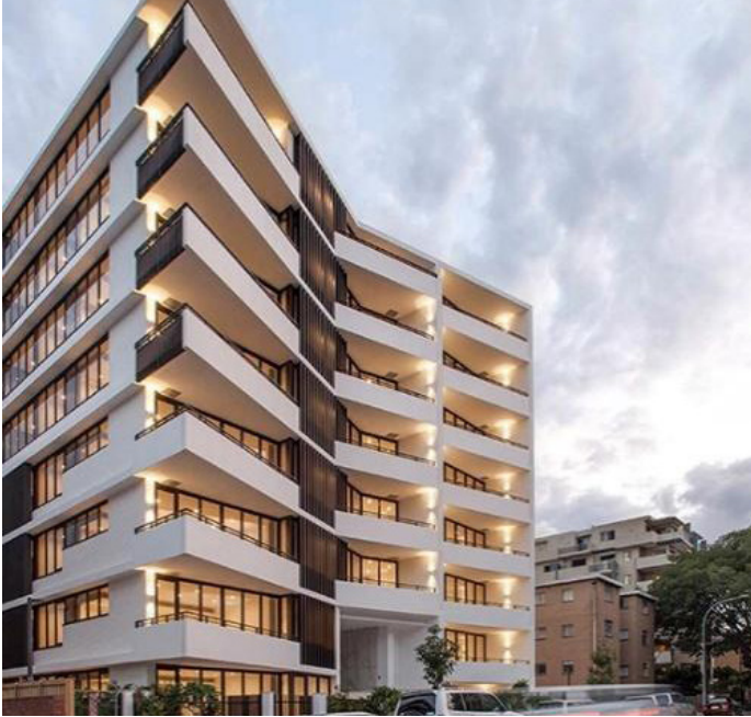
MIRVAC CONSTRUCTIONS The Moreton – Bondi Residential Contract Value $3,000,000
