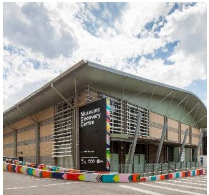
FDC CONSTRUCTIONS Power House Museum Castle Hill Commercial Development Contract Value: $1,500,000
