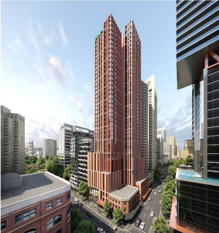
CPB CONTRACTORS Pitt St South Box Metro Infrastructure Contract Value: $6,800,000
