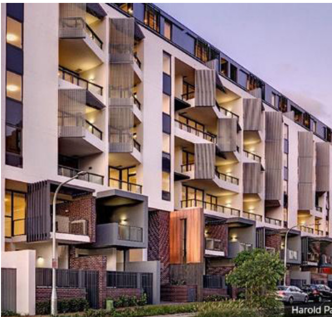
MIRVAC CONSTRUCTIONS Harold Park Precinct 6B Commercial & Residential Contract Value $1,200,000
